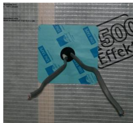
Figure 3.24 Air tightness grommet detailing for pipes and electrical services
