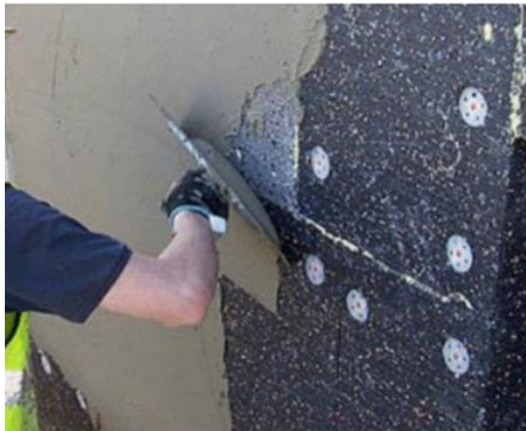
Figure 3.23 Plastering external insulation (Source: SEAI)
