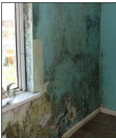
Figure 3.2: Surface Condensation leading to mould growth
