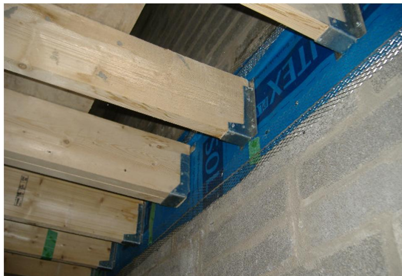
Figure 3.22 Wind tight membrane fitted at floor joist penetrations
