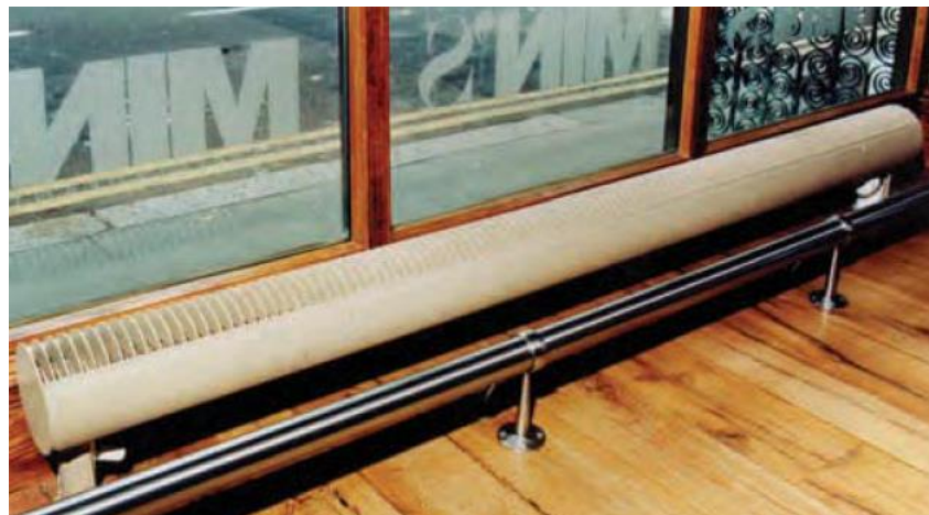
Figure 4.3 Compact low-level convector (Picture courtesy of Hudevad Ltd.)
