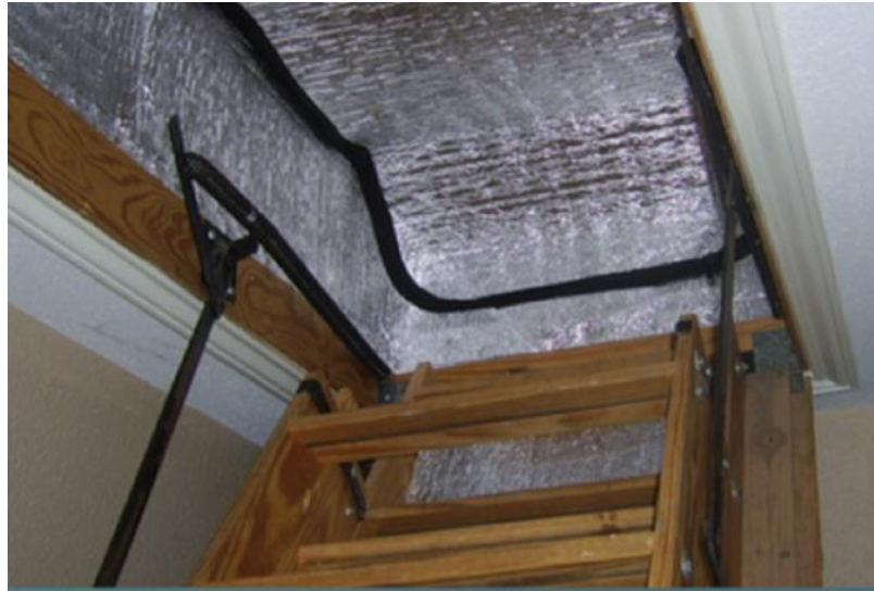
Figure 3.21 Airtightness tent to attic hatch
