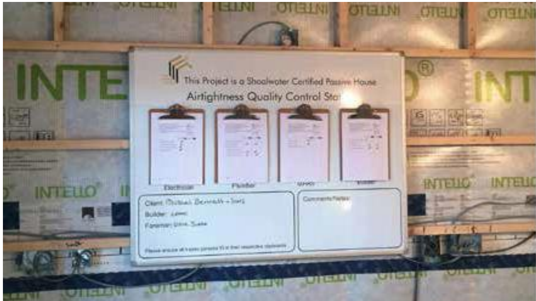
FIG 3.20: Recording air tightness testing at intervals to ensure compliance with NZEB
