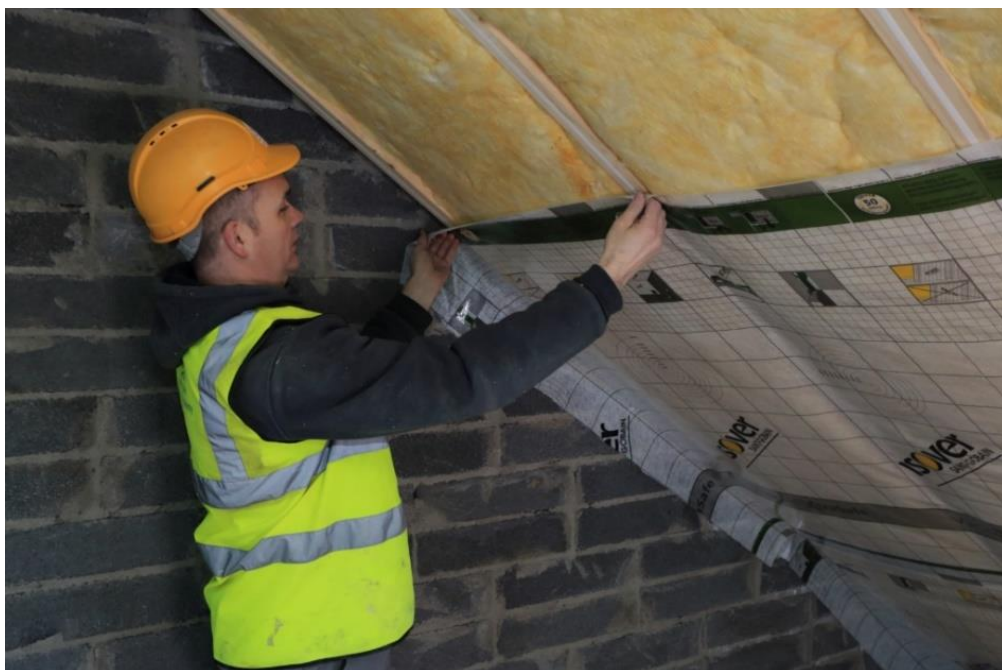
Figure 3.20 Air Barrier to underside of Rafter
